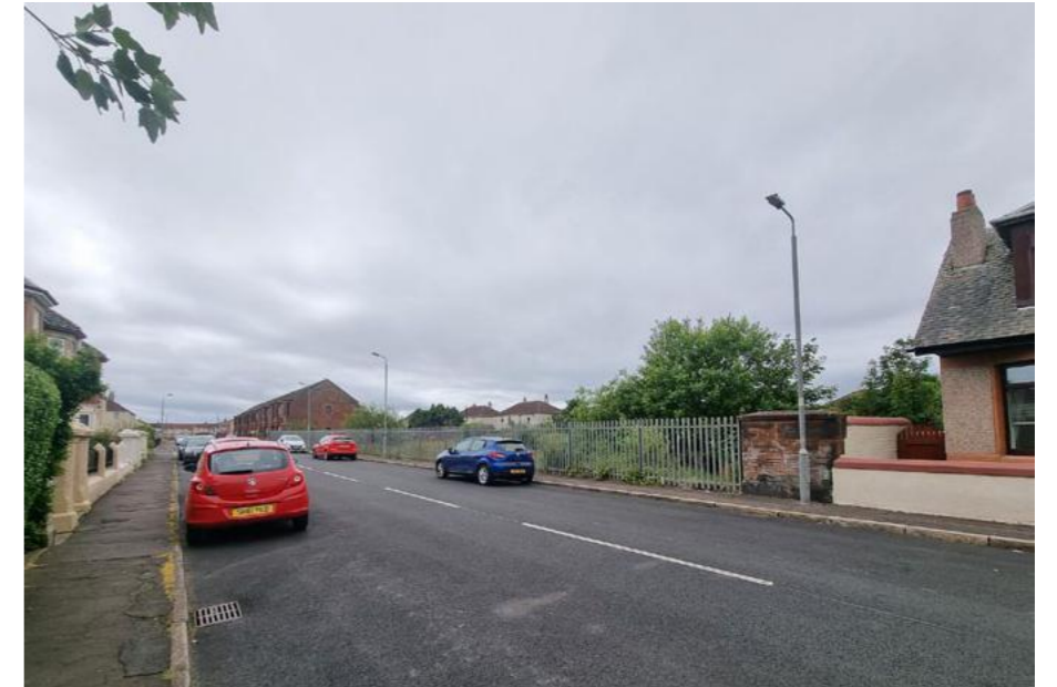
View of site on North approach from Garven Road
